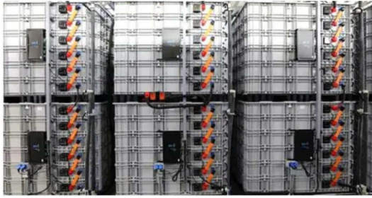
Tianning Lead-carbon BESS installation
