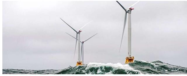
The first-ever electricity from offshore wind was generated at Vindeby. It's thermal sprayed zinc coating helped the wind farm survive six years longer than its intended lifespan – operating for 26 years and powering about 2,200 homes annually during that time.
